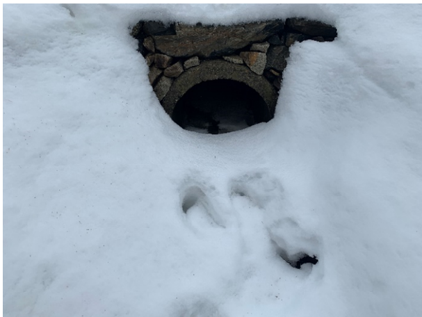
64 Gundalow - 1 (Drainage Course)
