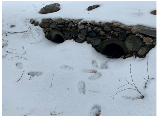
64 Gundalow - 2 (Drainage Course)
