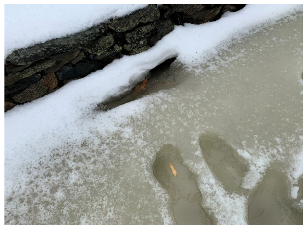
4 Brickyard Circle - 2 (Drainage Course)
