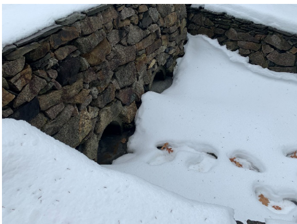
4 Brickyard Circle - 1 (Drainage Course)
